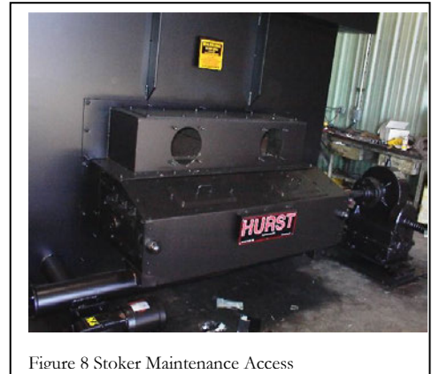
Figure 8 Stoker Maintenance Access
